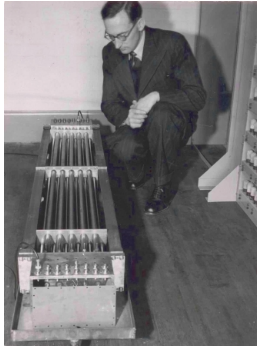
Memory Store: Mercury Delay Tanks
